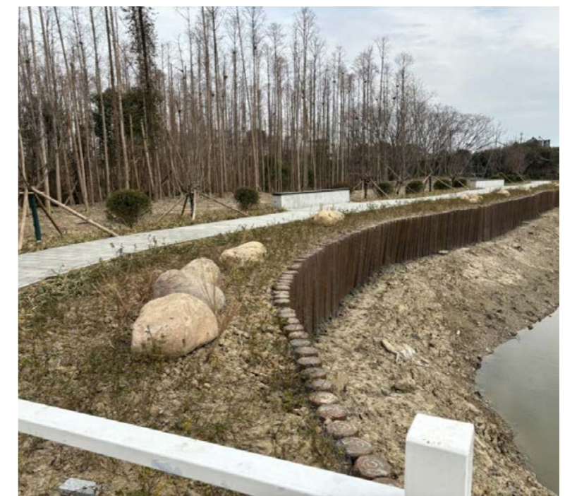
After embankment reinforcement in the Wangdian Interchange area
