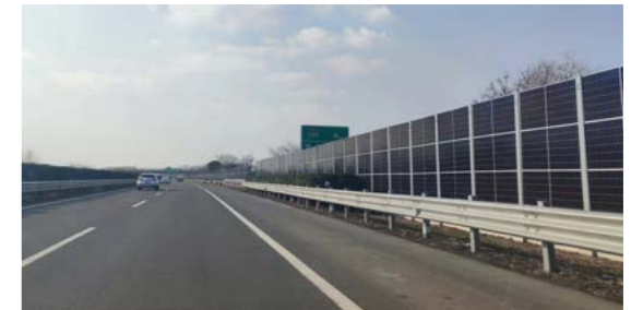
Shenjiahu Expressway sound barrier photovoltaic project
